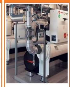
Building heat recovery chillers use ambient water to more efficiently produce hot and chilled water
