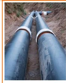
Underground ambient loop supplies temperate water to buildings at ~ 55 – 78°F
